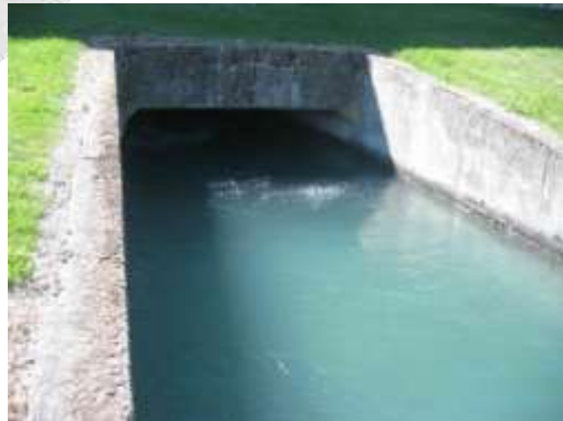
G8 tailrace after refurbishment
