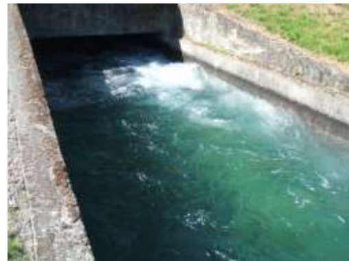
G9 tailrace before refurbishment
