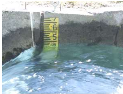
G9 weir height before refurbishment
