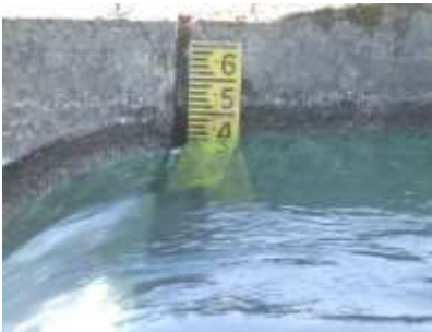
G8 weir height after refurbishment
